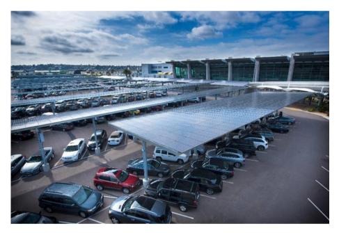
Results (Environmental Benefit/Cost Benefit): With the new solar photovoltaic arrays, SAN is annually generating approximately 9.3 million kWh of renewable electricity on site (about 20% of the Airport's total energy consumption).
