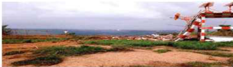
Photo 9: Broken ILS Mounting Structure Due to Impact of Wing
