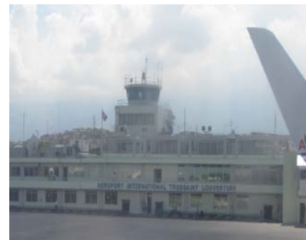
TOUSSAINT LOUVERTURE WAS DAMAGED SIGNIFICANTLY DURING THE EARTHQUAKE
