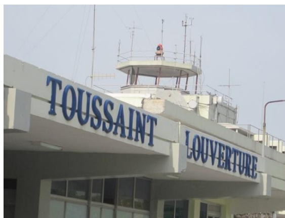
The major part of the country's main airport terminal was damaged beyond repair. Only a small area can be used for passenger handling.
