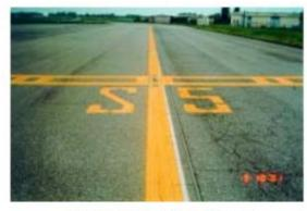
Photograph 10 - S5 marking and ICAO pattern B runway - holding.
