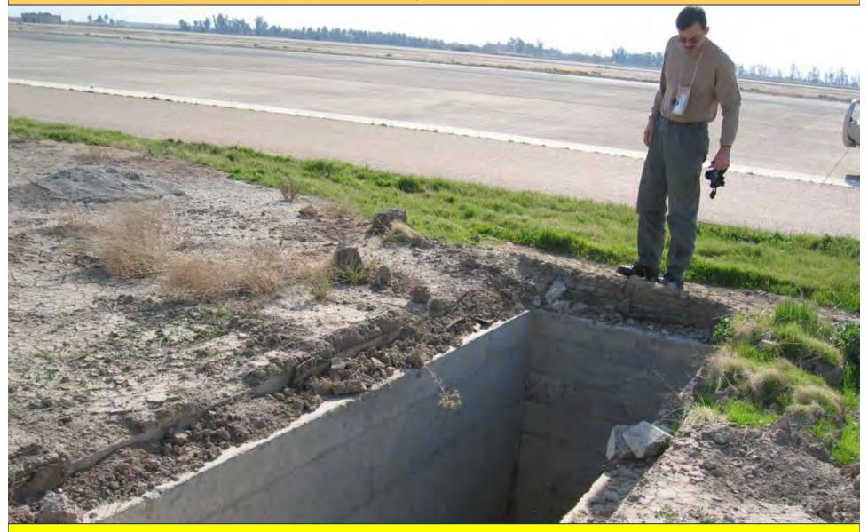
This open vault along the side of the runway is a significant safety hazard in the event of an aircraft running off the runway.
