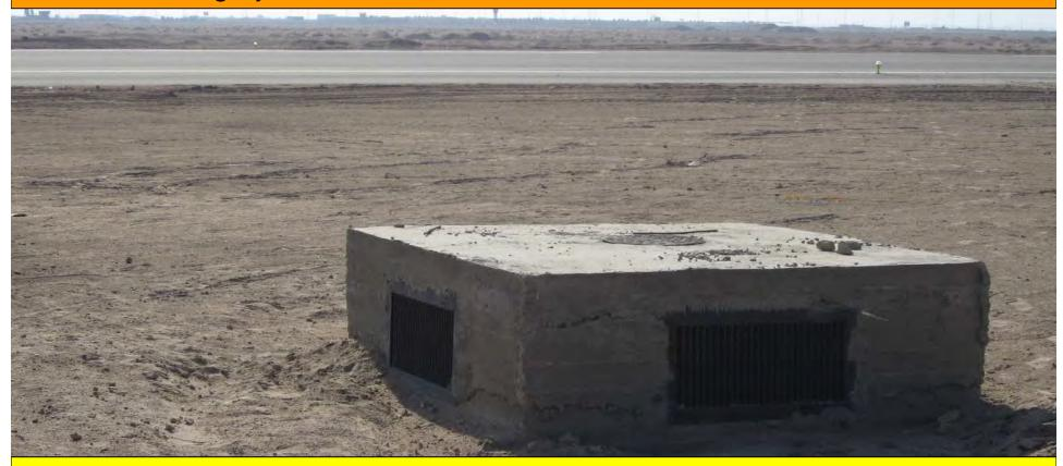
This large concrete structure provides a potentially hazardous situation in the event of an aircraft running off the runway.
