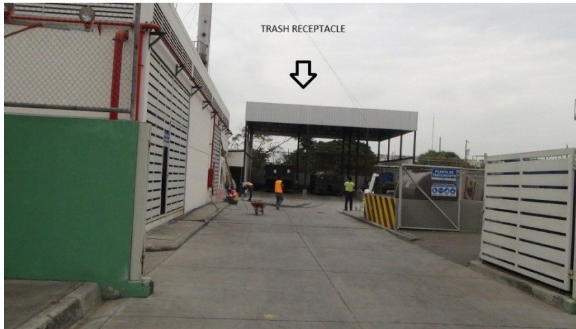
Trash Receptacles under covered structure
