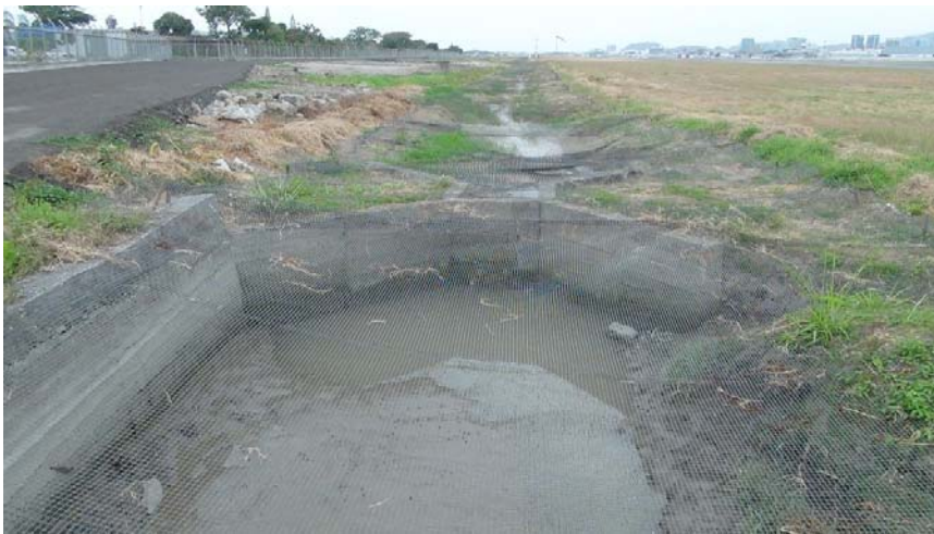
Large construction piles and mounds of dirt removed along canal
