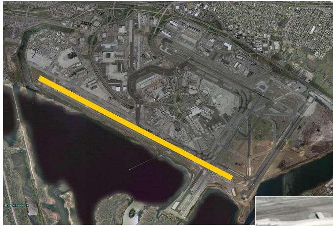
JFK Runway Reconstruction
