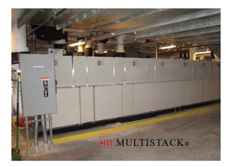
System uses 8 stacked heat pumps (up to 7 for cooling and all 8 for heating) to provide 100% of the terminal's cooling requirements and 75% of the heating needs
