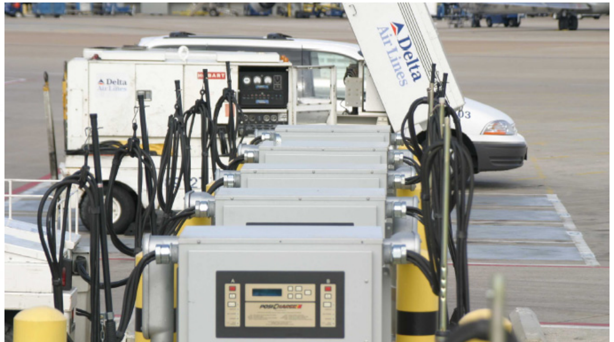
Rapid recharge station for Electric Vehicles at DFW
