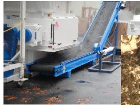
Shredding Cured CFRP
