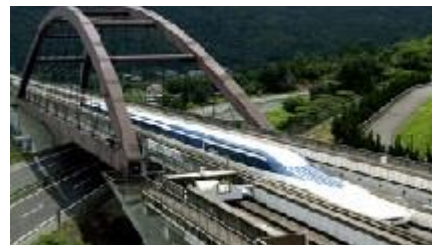
New Linear Shinkansen is under construction
