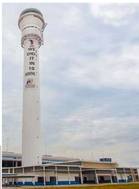
The tallest ATC tower (141.9 m)
