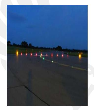
A series of unidirectional red lights, embedded in the pavement, right angles to the taxiway centerline, at the associated runway holding position, the lights are spaced 3 meters apart ,across the taxiway located 0.3 meters before the holding point lines.
