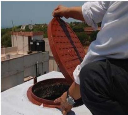
Figure 44. Mosquito-proof lid assembly of overhead tank © Ashwani Kumar
