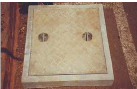
Figure 40. When closed this mosquito-proof lid assembly fits tightly on the margins of the service chambers © Ashwani Kumar
