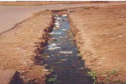
Figure 38. The wavy margins of the drain and floating plastic bags have created pockets where Culex species breed © Ashwani Kumar
