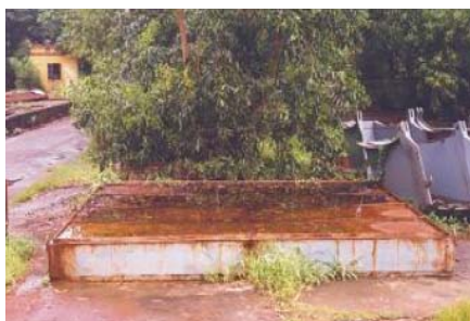
Figure 46. Iron platform with water © Ashwani Kumar
