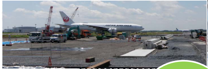
● Repair work & Expansion of facilities during operation
