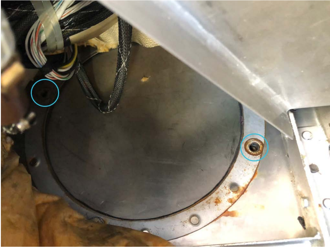
Figure 30: Magneto access panel on exemplar DHC-2 aircraft with two 4.76 mm diameter holes (circled) following bolt removal
