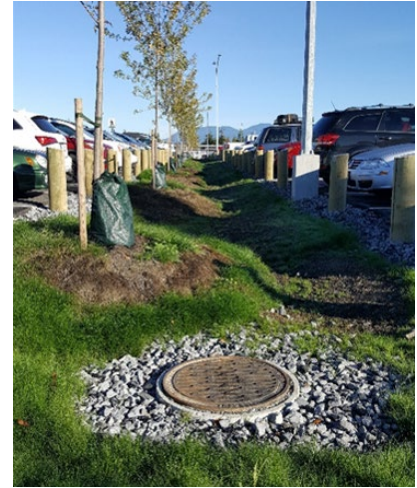
FIGURE 13: View of water filtering bioswale at YVR.
