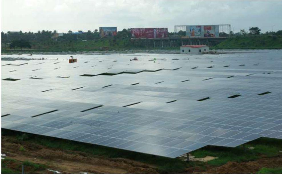
Cochin International Airport Solar Power Project is a 40 megawatt (MW) photovoltaic power station
