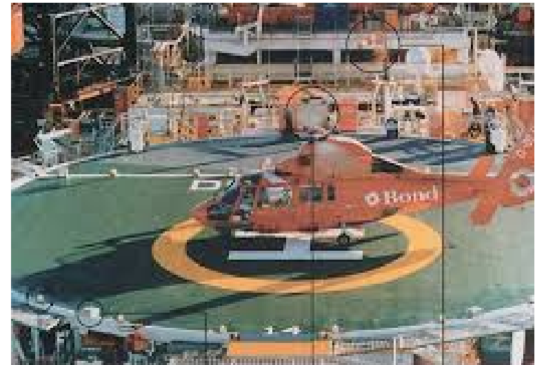
Perimeter light yellow Floodlight for 8:1 illumination uniformity ratio Ground Power Unit (helicopter starter) inside illuminated wind sock
