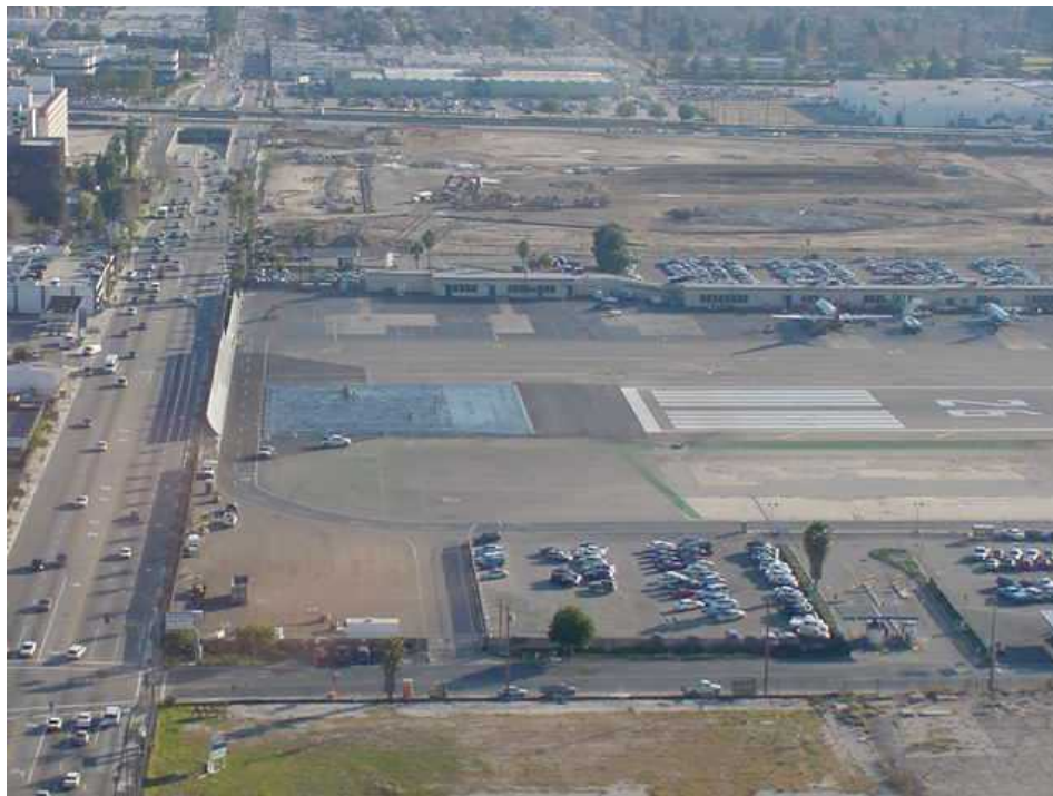
Figure 6 - Aerial photo showing (a) relationship of Hollywood Blvd. off Runway 26 at Burbank Airport, Burbank, California and (b) EMAS installation awaiting chevron-markings
