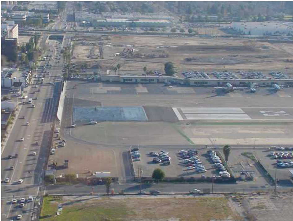
Figure 6 - Aerial photo showing (a) relationship of Hollywood Blvd. off Runway 26 at Burbank Airport, Burbank, California and (b) EMAS installation awaiting chevron-markings
