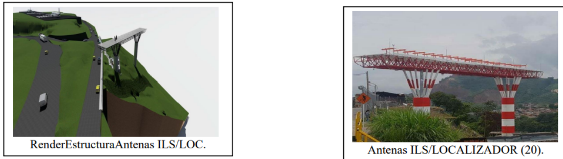
Figure 1. ILS LOCATOR Antenna System
