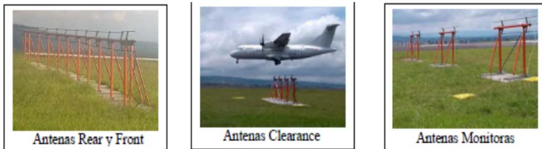
Figure 2. ILS/GLIDE PATH Antenna System END FIRE Watts Antenna
