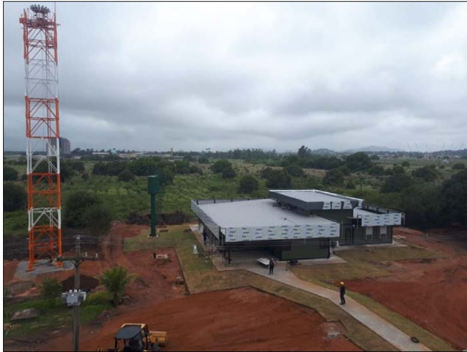
Figure 1 - Facilities of R-TWR Santa Cruz
