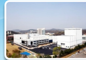
KASS Control Station
