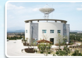
KASS Uplink Station
