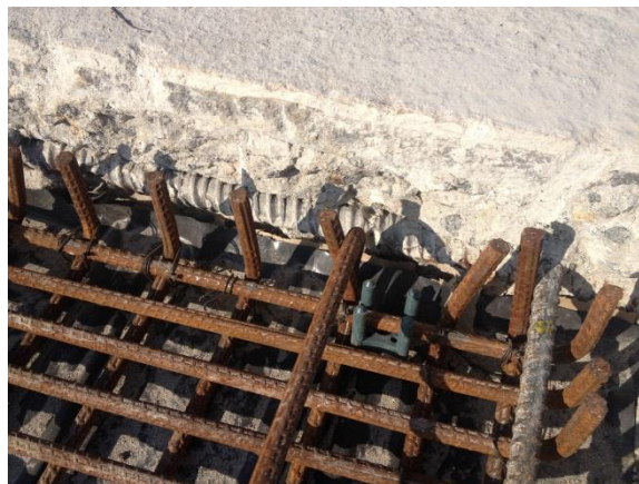
RWY panel being repaired
