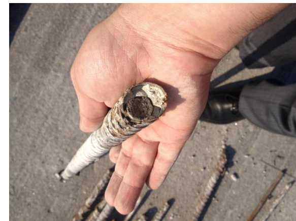
RWY panel being repaired
