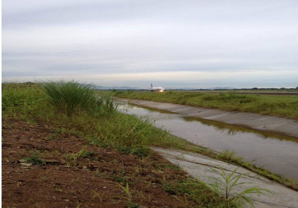
Concrete-lined canal next to runway
