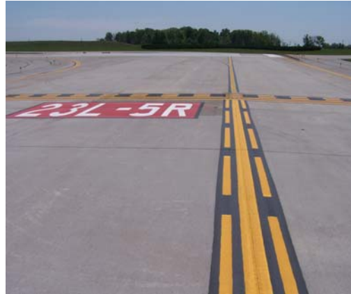
Enhanced Taxiway Centerline Markings
