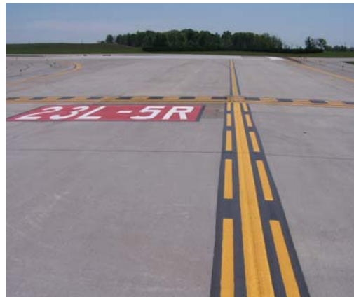
Enhanced Taxiway Centerline Markings
