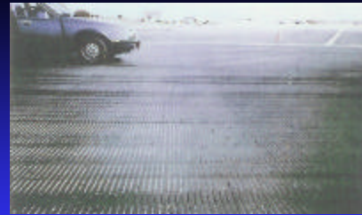
Fig.6- The grooved asphalt surfacing on Runway 13L-31R, at J.F.K. Airport, photographed after a year of service.
