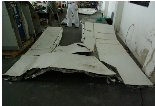
Figure 39: Ceiling of the LDMCR: with top-downwards deformation
