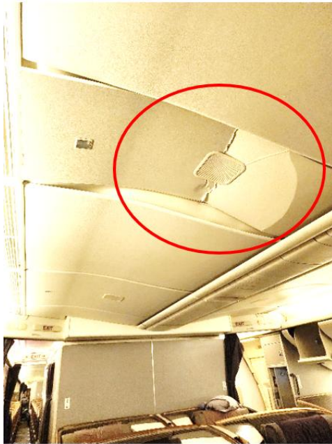
Figure 4: Broken ceiling panel
