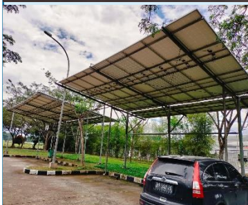
Solar PV at Parking Area Kalimarau Airport, Cap. 360Kwp Operated on Dec 2016
