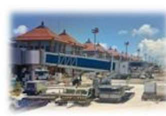
LED for apron flood light
