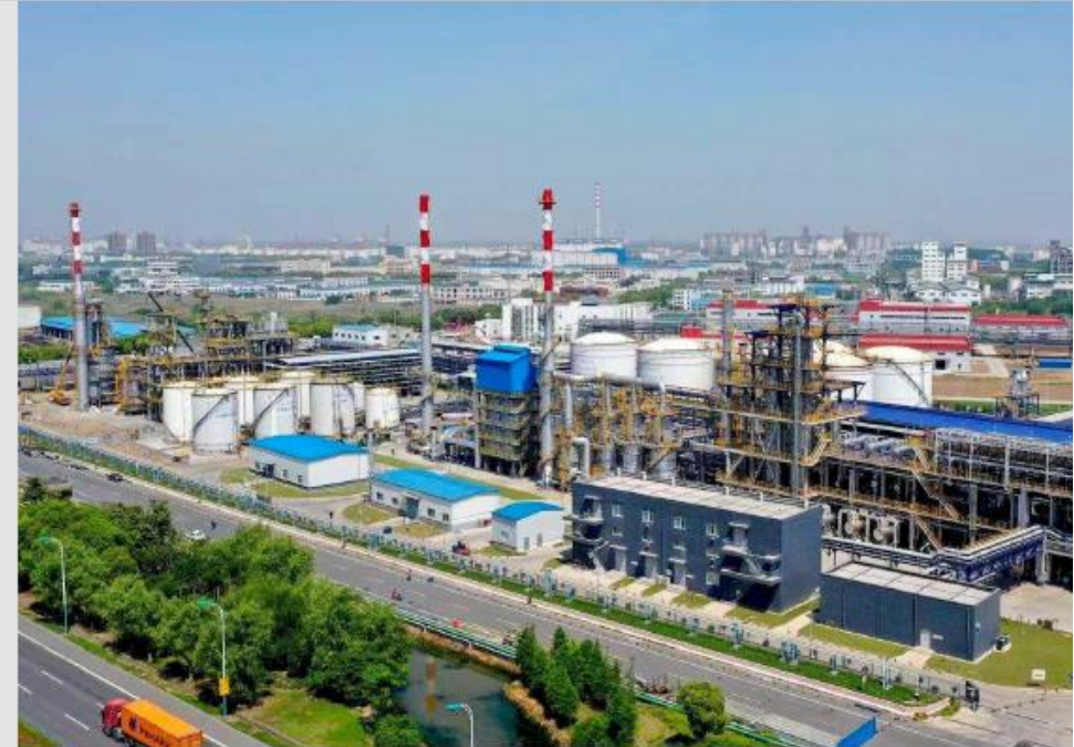
SAF/HVO production facility in Jiangsu, China
