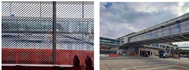
FIGURE 3: Advanced screen-printed glazing installed.
