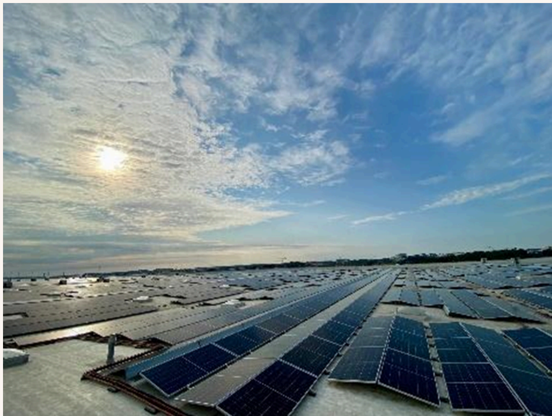
Figure 7. Brussels Airport Cargo: A new installation of 65.000m 2 of solar panels (7.3 MW) covering the roof of our newest building at Brucargo.
