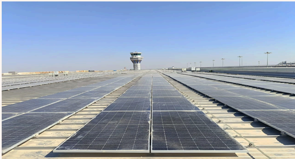
Figure 9. Borg El Arab International Airport – Solar farm on the terminal phase 2 with capacity 1.4 Mw
