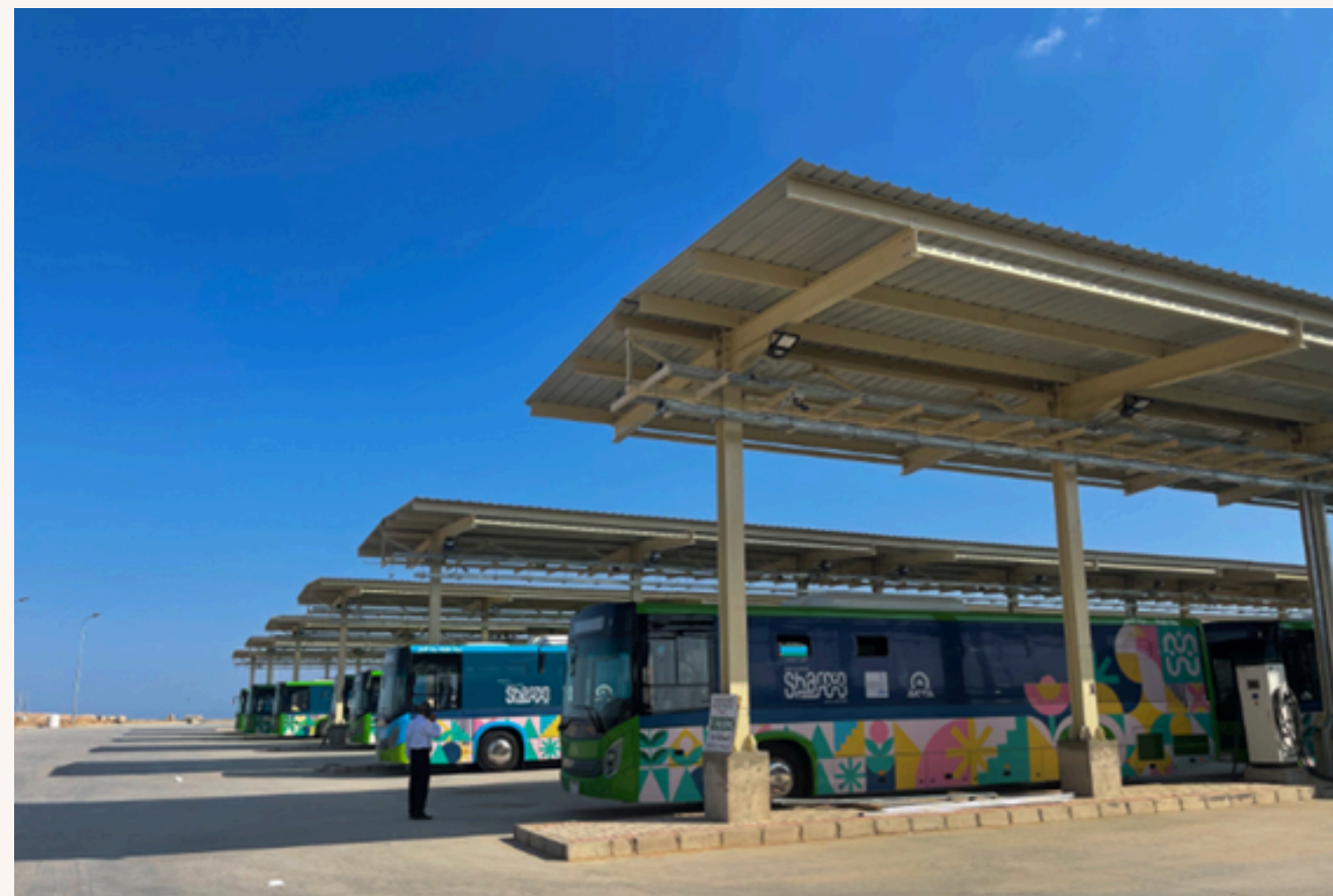
Figure 10. Sharm-El Sheikh International Airport – Electric buses
