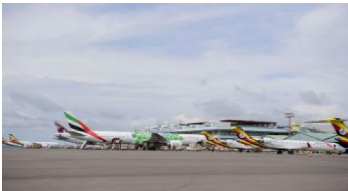
Entebbe International Airport
