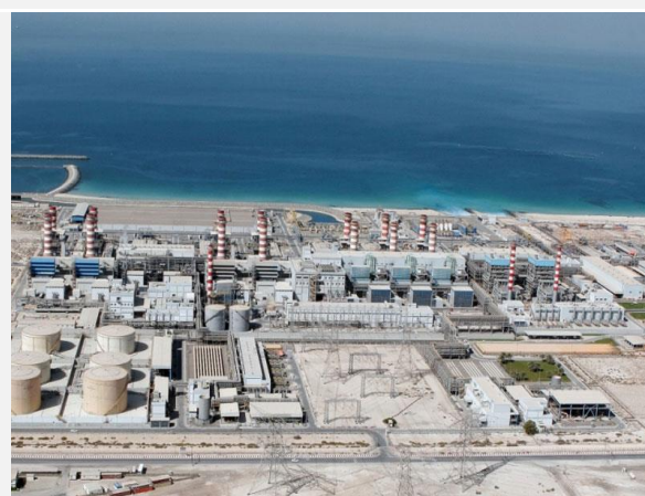
Figure 31. For reference, the world's largest desalination plant, Jebel Ali Power Plant & Desalination Complex in Dubai, UAE, can desalinate 2.2 million m 3 per day. 105
