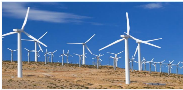
Figure 27. Tafila Wind Farm, Jordan's largest wind farm with a capacity of 117 MW, currently covers roughly 2% of Jordan's electricity demand. Operational since 2015. 102
