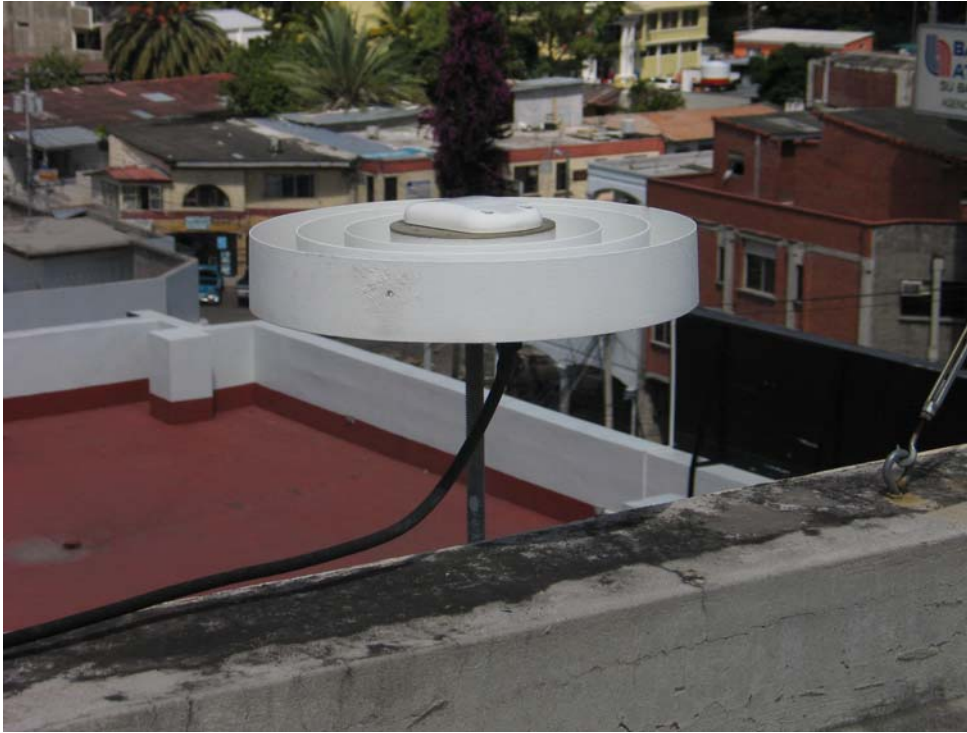
GPS Antenna Tegucigalpa Honduras
