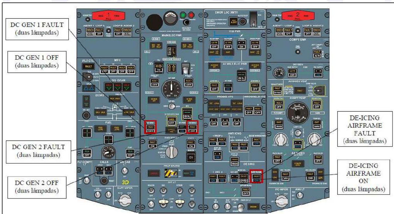
Figure 76 – Overhead panel showing the positions of the indicator lights from which the lamps were removed for examination.
