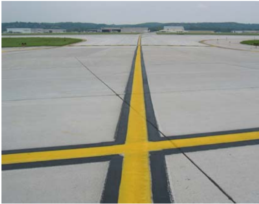
Previous Taxiway Centerline Markings
