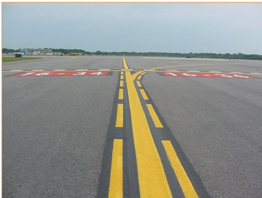
Enhanced Taxiway Centerline
