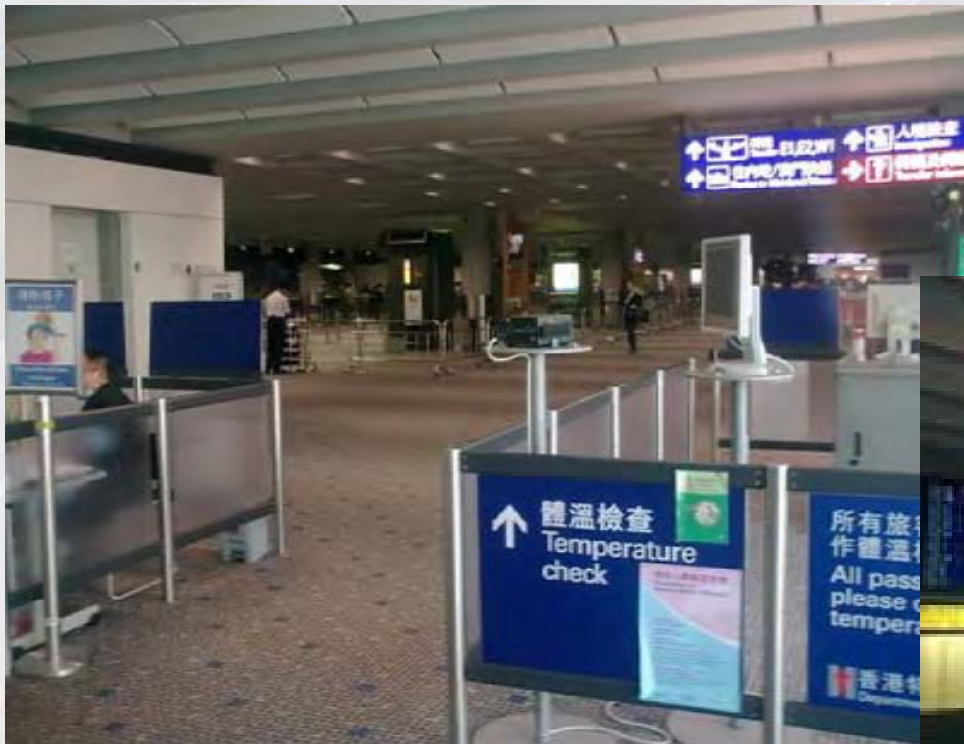
↳ Thermal infrared scanning system / base mounted
