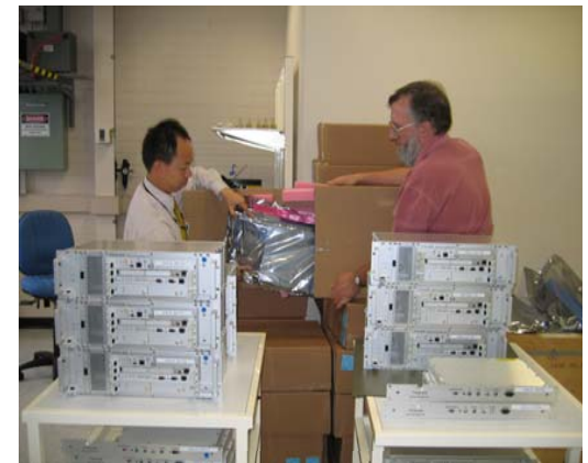
GROUND STATIONS ARE BEING INSTALLED
