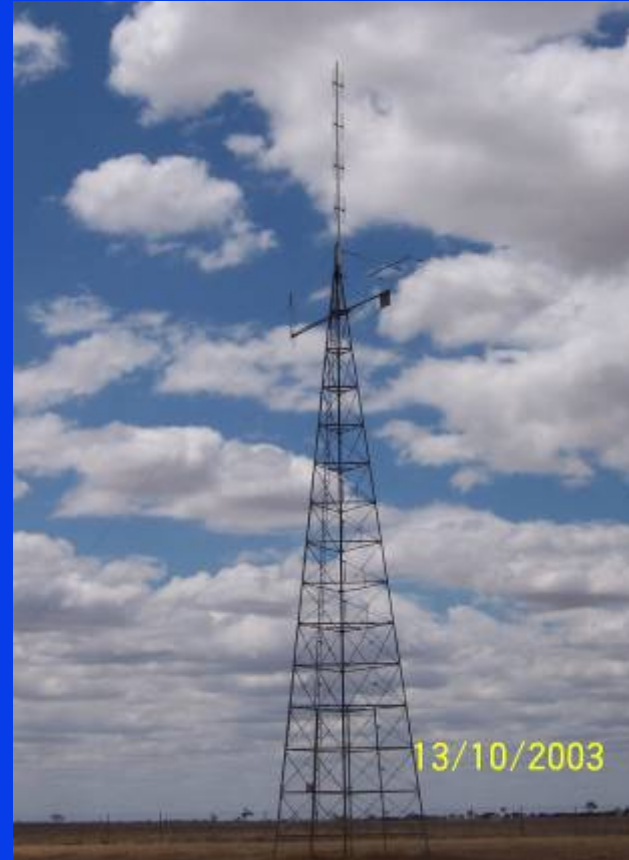
Tower replacement project!
