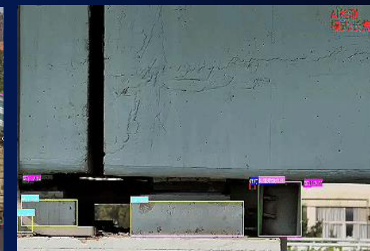
Traffic Quality Inspection
