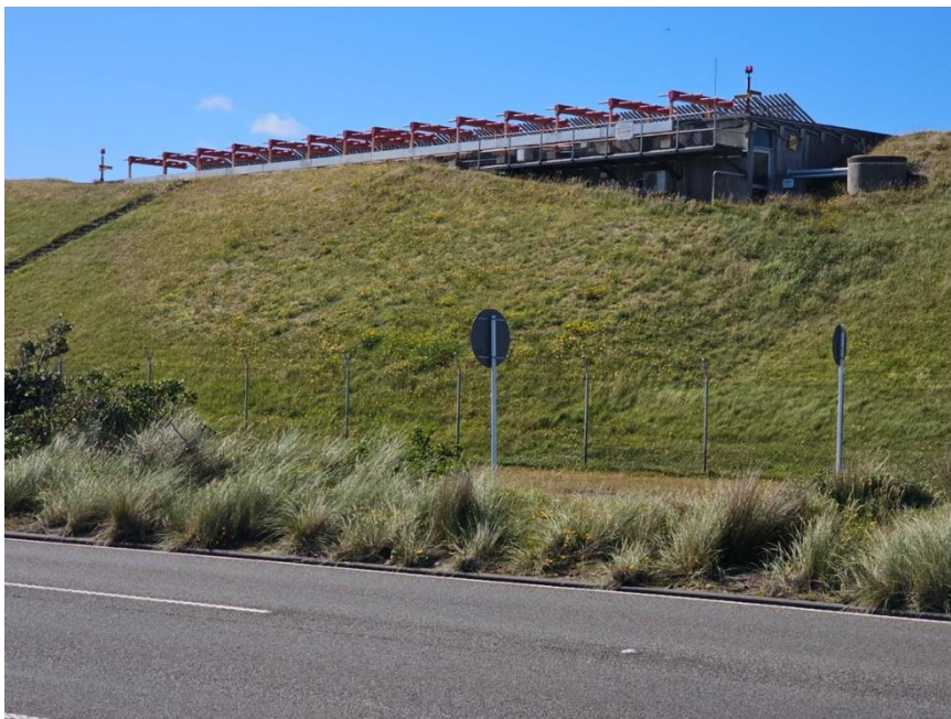
WLZ – LLZ (Localizer) bunker
