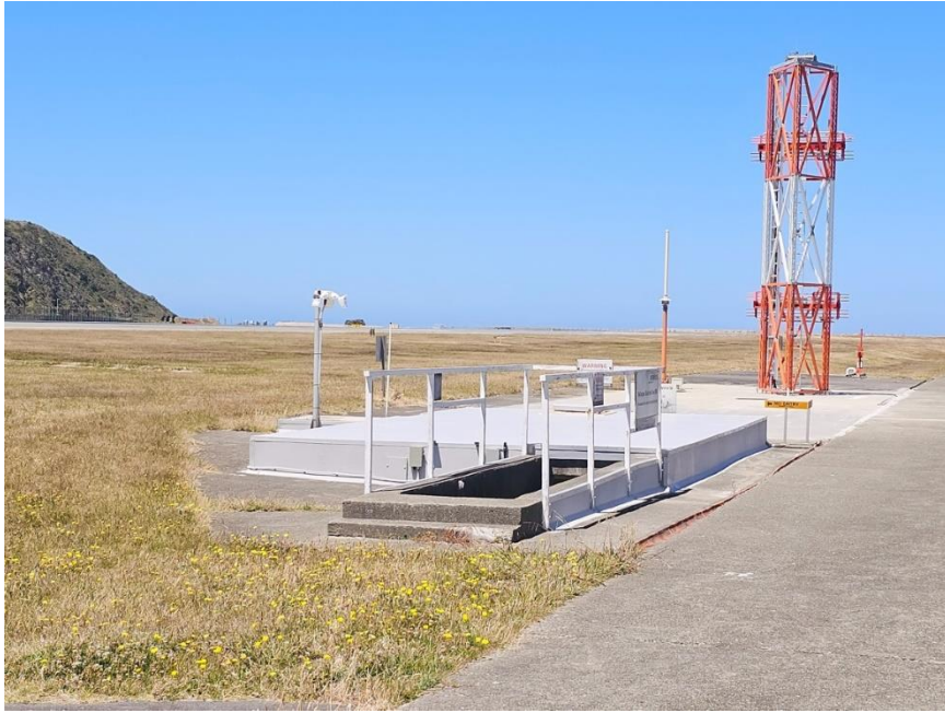
WLK - Glidepath Bunker
