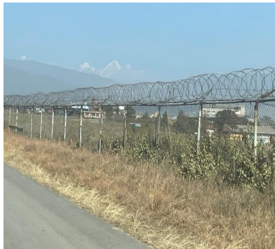
Figure 3: Non-Frangible security fence
