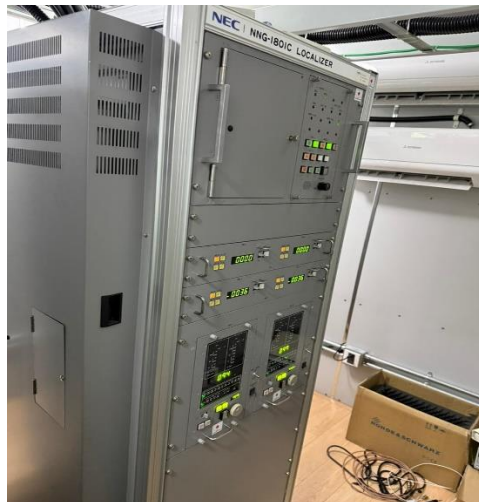
Figure 5: ILS Hut with equipment
