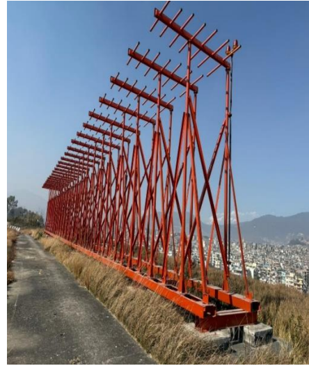
Figure 4: ILS / Glide path antenna and equipment on the runway strip
