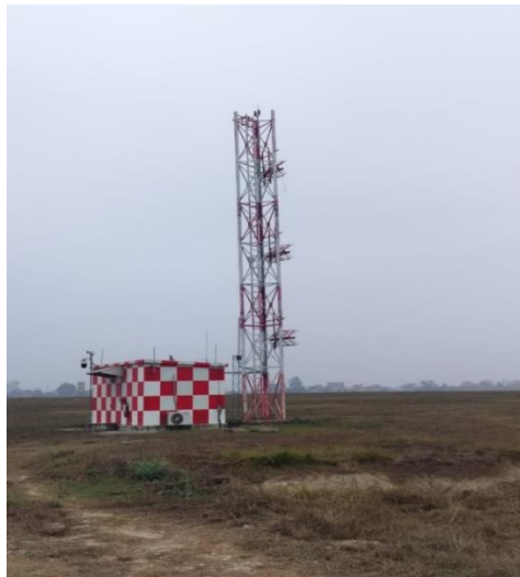
Figure 4: ILS / Glide path antenna and equipment on the runway strip
