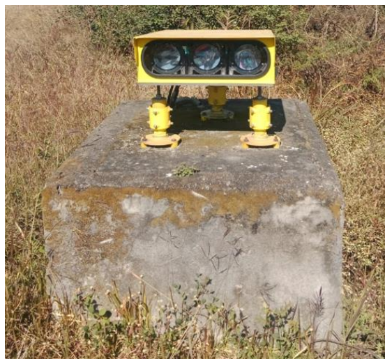
Figure 1: Elevated foundation of PAPI on the runway strip
