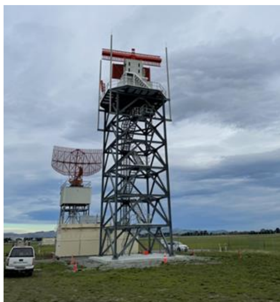
Fig. 1 - New NZCH MSSR/PSSR in front of the old PSR
